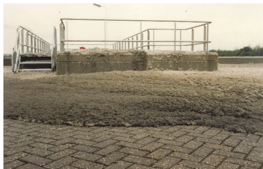
Figure 10.11 Extreme manifestation of sludge bulking (photos: Eikelboom, 2006).
