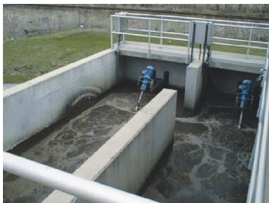
Figure 10.7 Aerobic selector (photo: M. van Loosdrecht).
